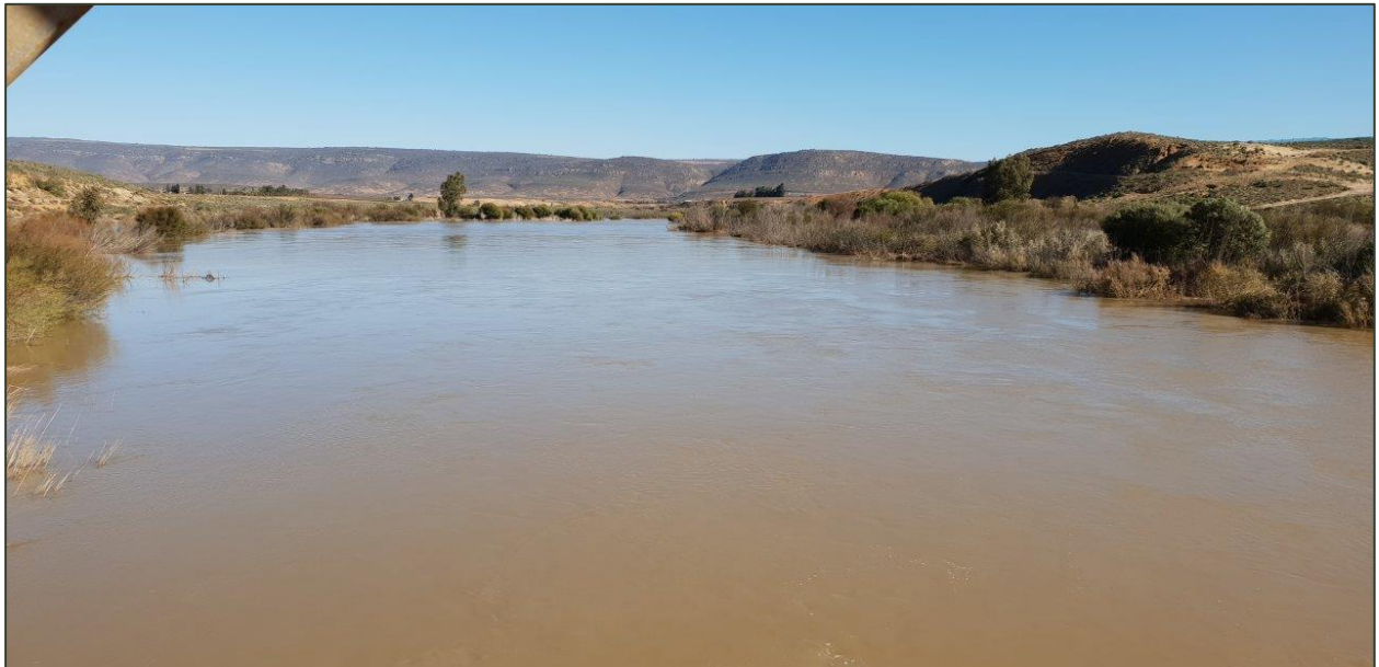
Figure 5.10: Photo taken at the proposed siphon location through the Olifants River while the river was in flood during July 2020
